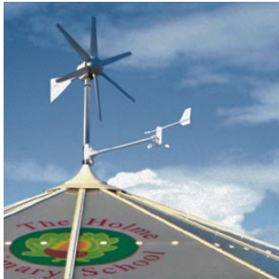
Environmental Shelter with weather station and wind turbine
